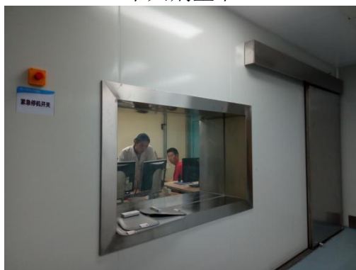
机房内紧急止动按钮
